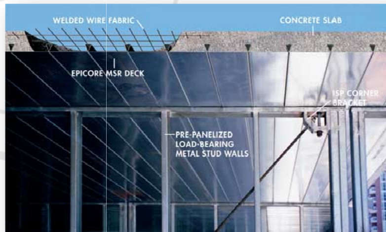
Figure 22.A: Epicore MSR Composite Floor System (www.infinitysystems.com)
