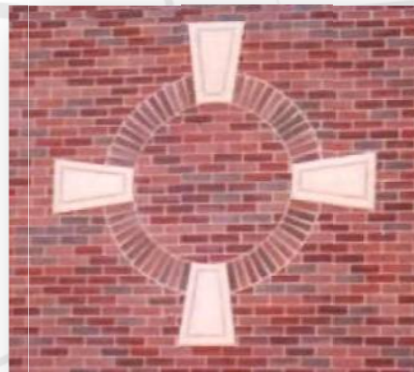
Figure 2: Thin Brick Precast Panel (API Manufacturer: www.apiprecast.com )
